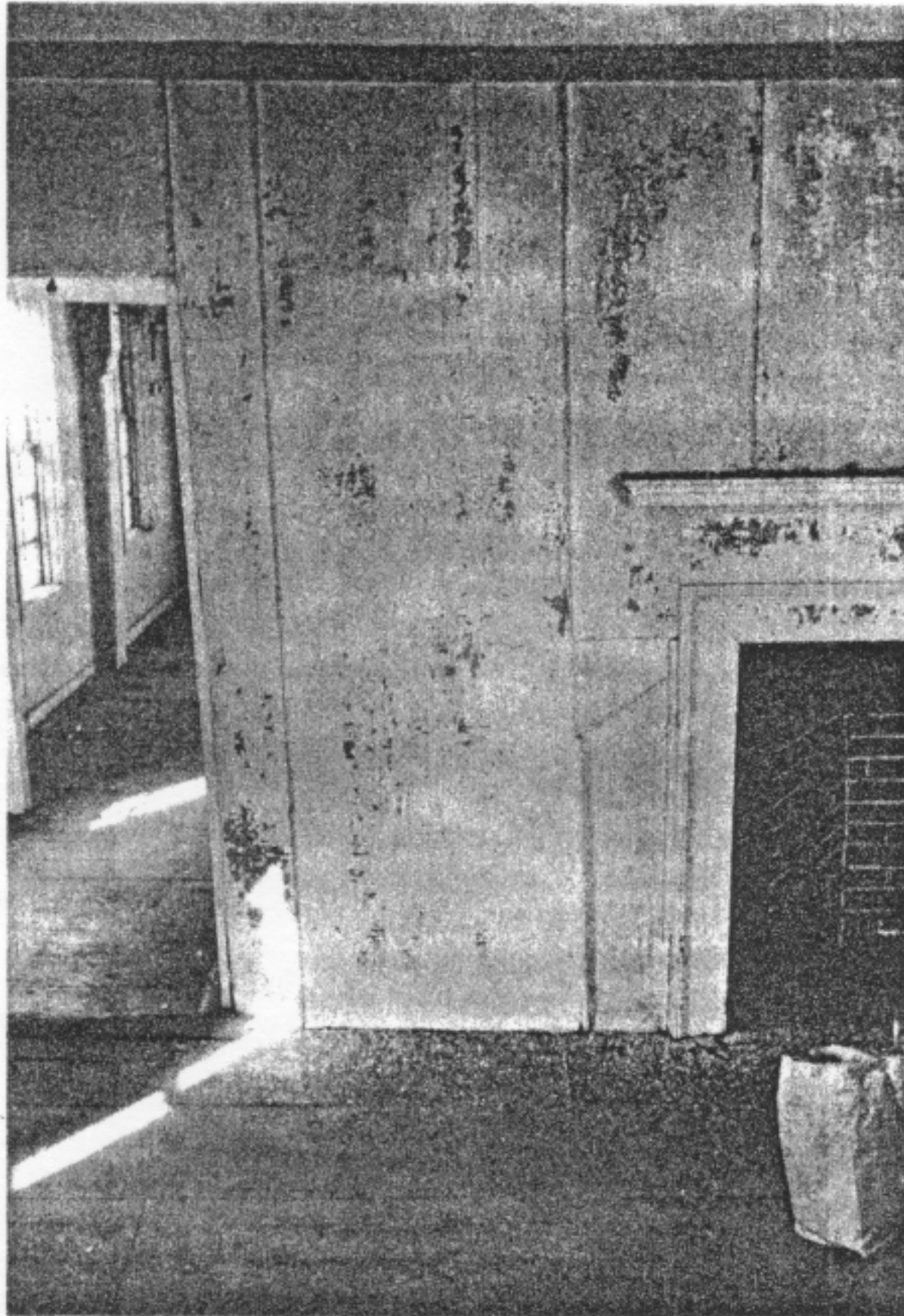
Fig. 21 South chamber, second floor. Area examined for evidence of stud mortices is floor just to left of fireplace.
